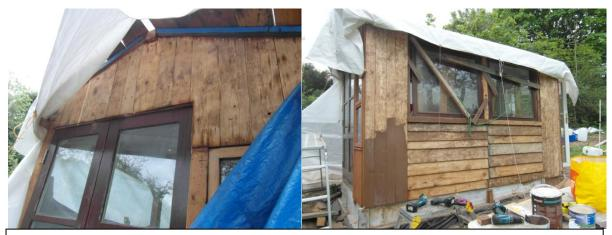
The cladding is going onto the frame, sanding the old wood stain ahead of giving 2-3 coats of Acorn Gold and Slate Grey....purchased from Hunts closing down sale.
