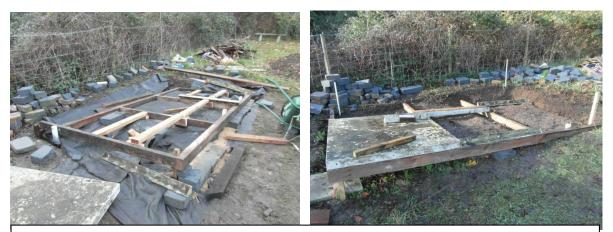
The new shed Base needed soil to be dug out and Framework supported on Legs to offset the Slope of Orchard. used mix of reclaimed roof timbers and donor floor joists. Base also used 4ft x4ft 4ft x 2ft Glass Fibre glass panels to clad and weather-proof base.
