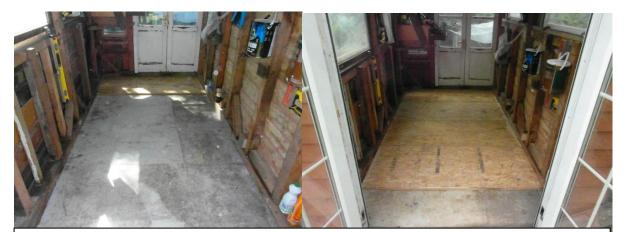
Inside of shed floor: Fibre Glass panels (very Flexy despite being 1cm thick) ...I decided to cover in 22mm OSB Board from Reclaimed Timber (Maidenhead) qty five needed. (each board 6ft x 29inches wide to cover 12ft x 6 ft floor area, consequently additional cost is 5 x £5:00 each (6ft long x 29inches wide) = £25.00
